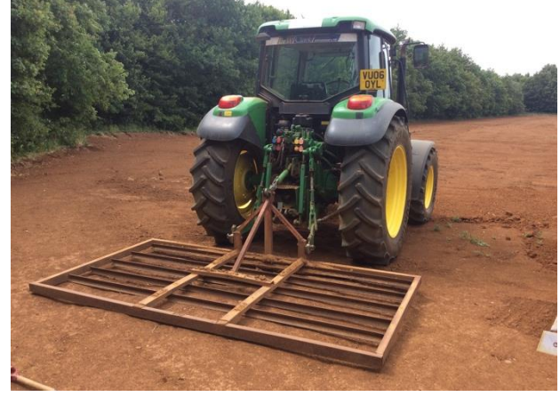
Figure 12: A final rough grading with the levelling bar will eradicate any surface imperfections and iron out the minor mounds and depressions detailed above.
