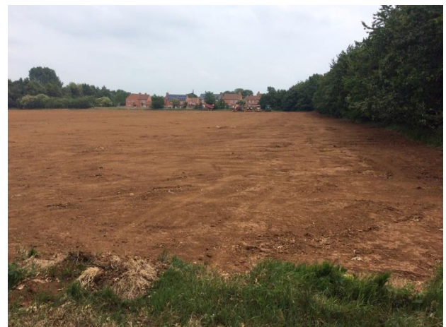
Figure 10: A section of the site immediately adjacent to the road at the south end of the field has been stripped, roughly graded and compacted in preparation for the construction of facilities and car-parking.
