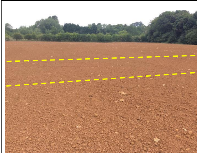
Figure 7: A slight was evident through the centre of the site for pitches from West to East, particularly towards the eastern boundary. Final cultivation and levelling should aim to correct this prior to drainage installation.
